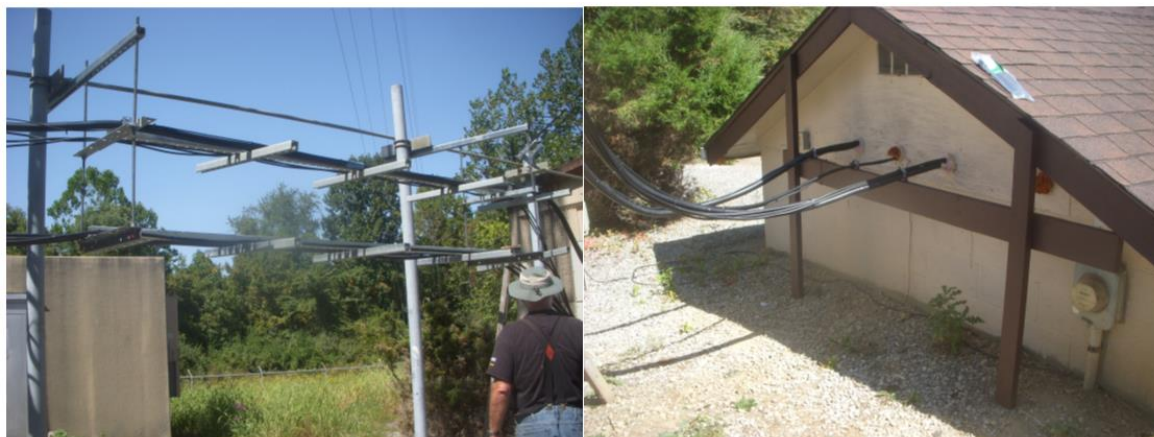
New Ice Bridge and building cable entry
