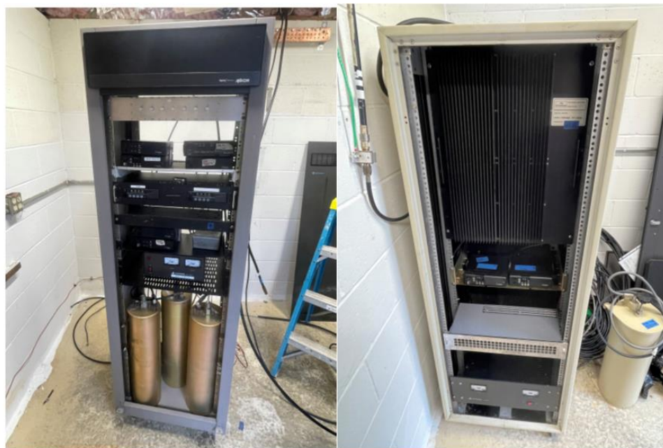
New cabinets for receivers ('16, '37, '93, 6M) on the left and '33 transmitter on the right.
